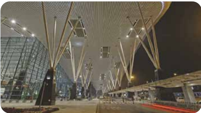
Airport - Madurai, Ayodhya & Delhi Terminal 1
